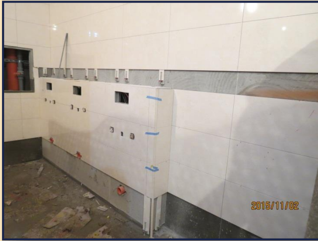
廁所牆面磁磚安裝
